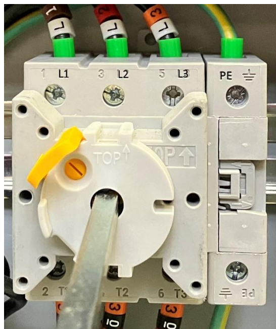
Figure 7 - Electrical connection of the machine
